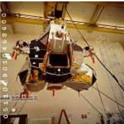
**Lunar Module 5 ascent stage in Final Assembly area on overhead hoist.**
